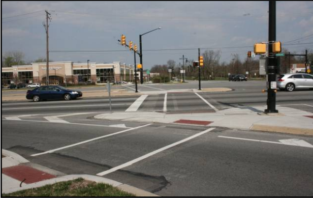
West Whiteland Township, PA: Example of a pedestrian crossing across a busy section of Route 100. This example shows well marked crossing design a safe area between the right turn lane and flow of traffic.
